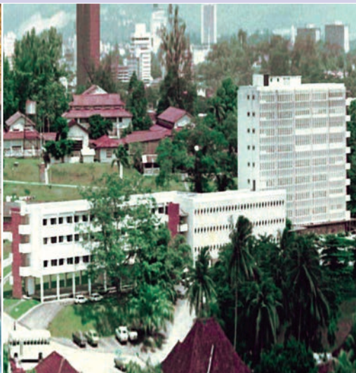
IKU building in the early days with Bangsar Hospital in the background
